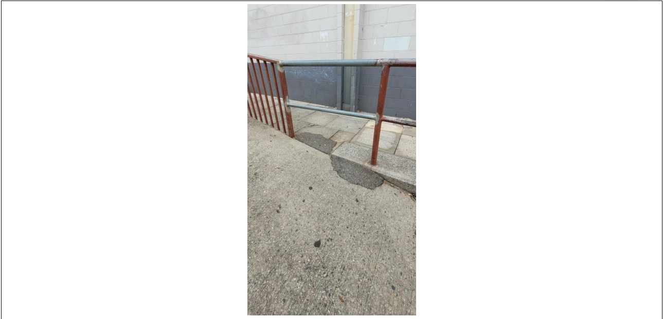
Figure 8: Retained bitumen at the abutment between the slab path and steep ramp, railing in situ
