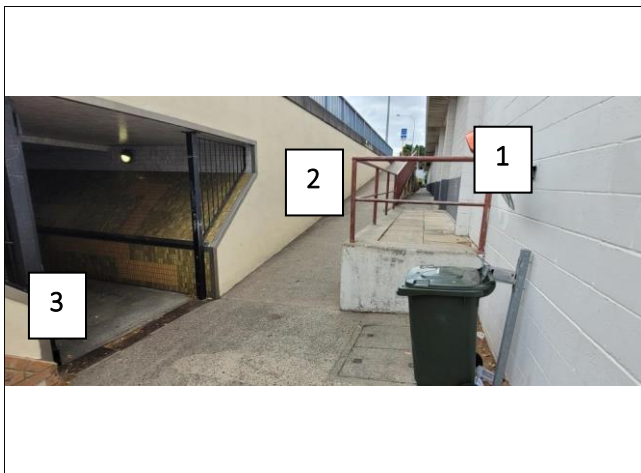
Figure 4: End of slab path [1], ramp [2] & underpass [3]
